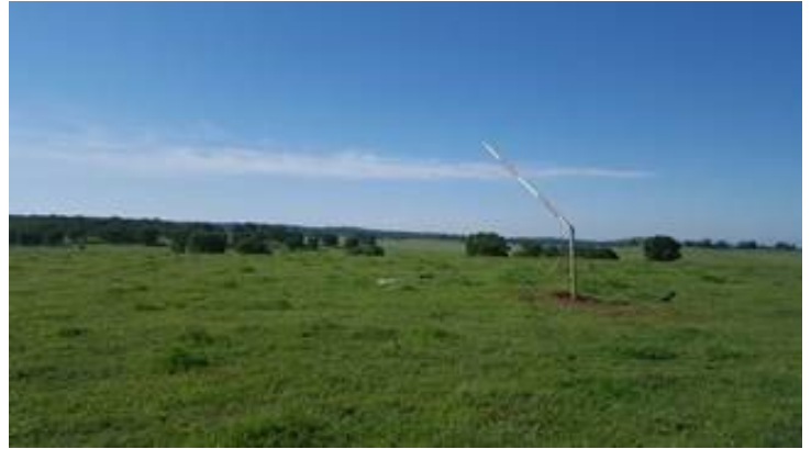
This is the west pylon after the collision.
